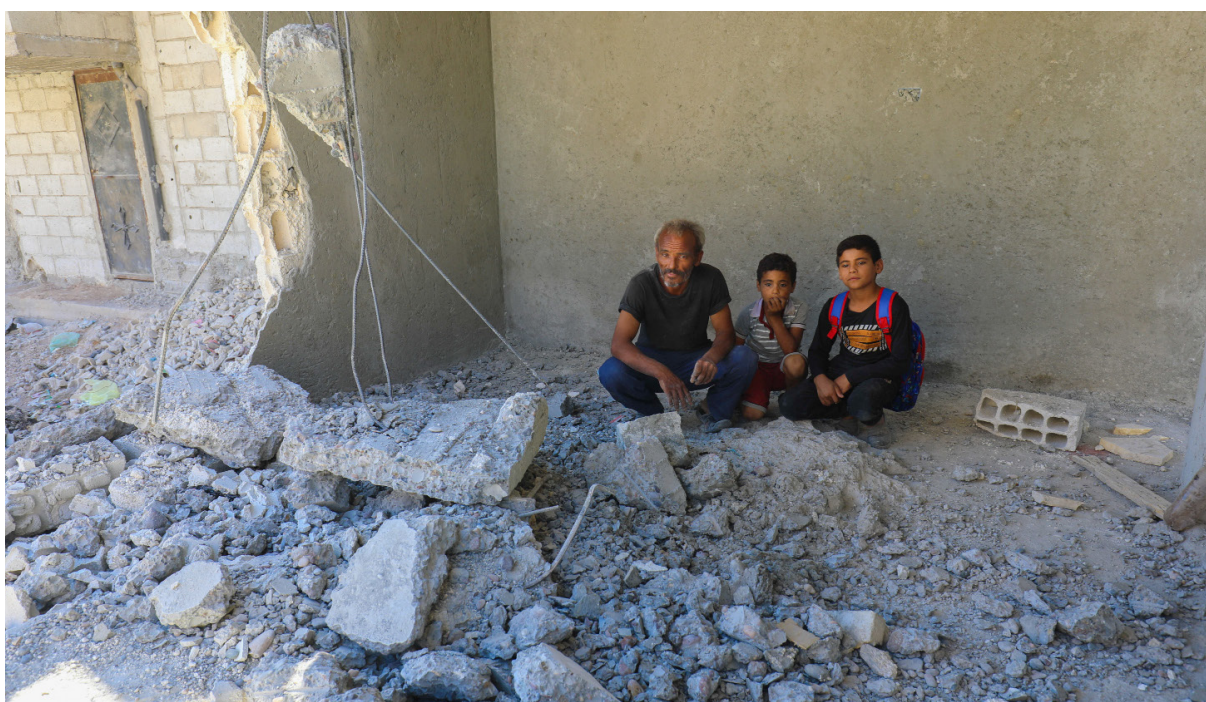
Yaseen* is 12 and is currently living in a building site with his family. Photo taken by Muhannad Khalid, Save the Children.
